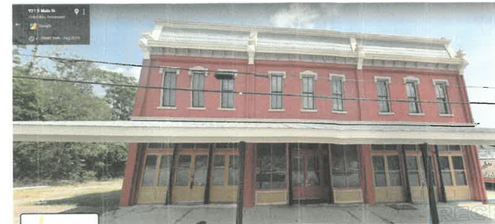
ADJACENT BUILDING TO THE RIGHT OF PROPOSED.
