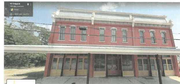
ADJACENT BUILDING TO THE RIGHT OF PROPOSED.
