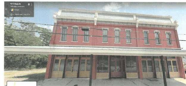
ADJACENT BUILDING TO THE RIGHT OF PROPOSED.
