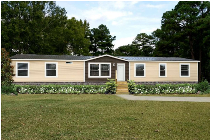
PHOTOS TAKEN FROM HAMILTON HOMES https://www.hamiltonhb.com/our-homes/
