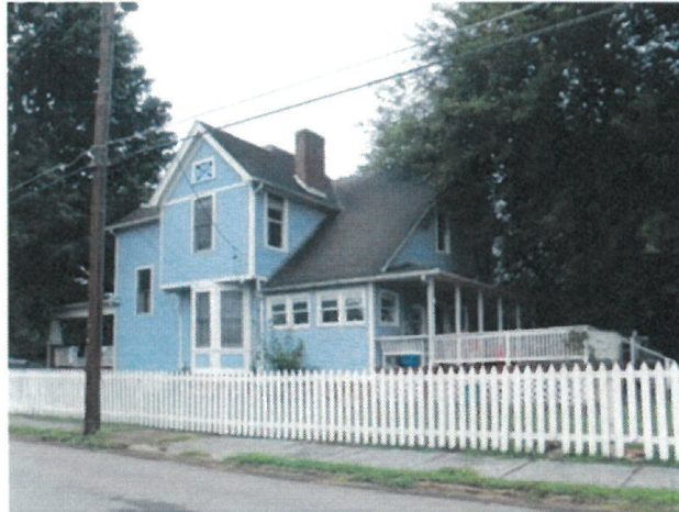
LOCATING DECKS Decks should be appropriately scaled to the house and screened from view along the right-of-way when located on a visible elevation. Decks that are overly large and visually prominent such as the one in the above photograph detract from the character of the building and streetscape, draw unnecessary attention, and are not appropriate.
