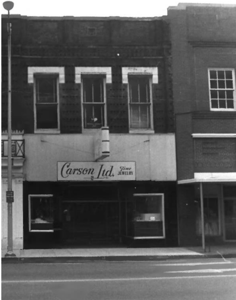
118 West 7 th Street as it appeared in March 1984
